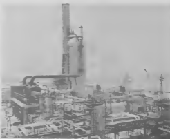
Vacuum Pipestill with HDS Process Stack.
